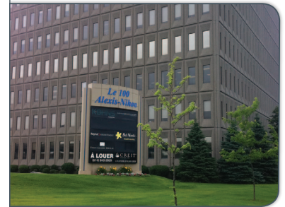
Montréal, Quebec facility
