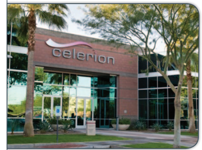
Phoenix, Arizona facility
